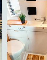
MOBILE & TRANSPORTABLE FACILITIES
